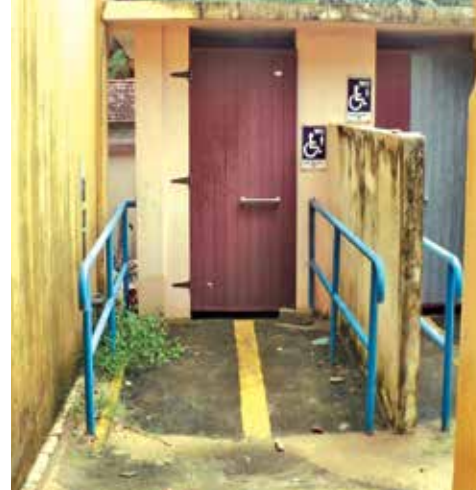
The yellow line on this access ramp to a latrine helps to guide a person with visual impairment
