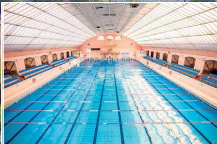
Swimming Pool of the Central Command of the Armed Forces of Ukraine after reconstruction. 2005
