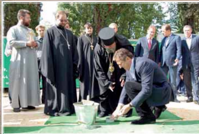
Laying a capsule at the construction site of the sports complex «Liko»
