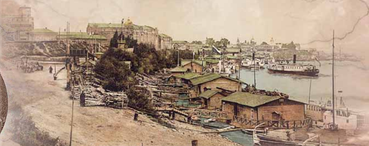
Kyiv. Dnipro River embankment near the aquatic centre. Early XX century
