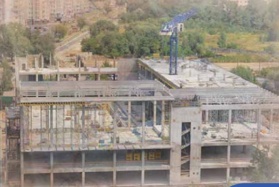
Construction of one of the best high-tech pools in Europe - «Liko»
