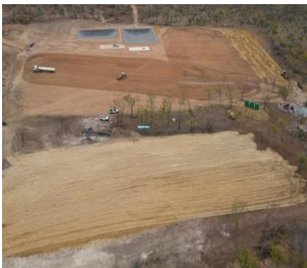
Fig. 5. Photograph of the Mukuyu-2 well drilling site [1].
